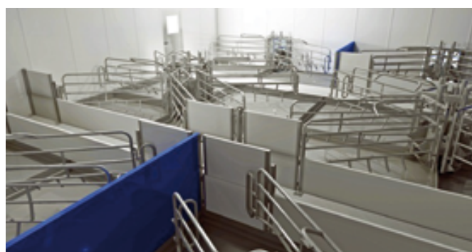
Delivery room before grids are put in place.
