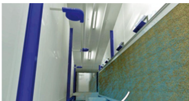
Ventilation inlets lower cellar trays.
