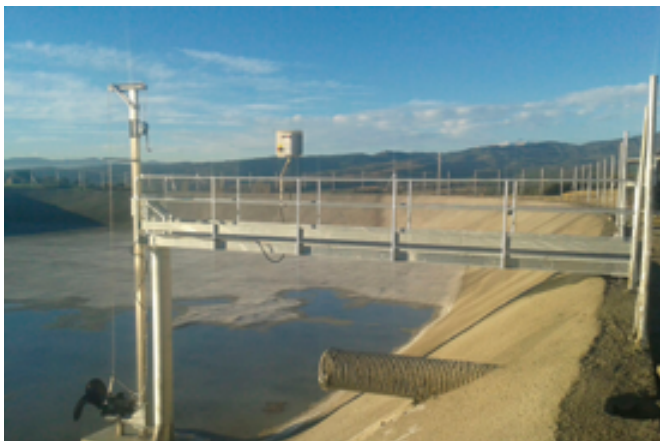
SUPPORT FOR SLOPE RAFTS WITH INTERNAL SUPPORT For newly constructed basins, with concrete or PVC slope
